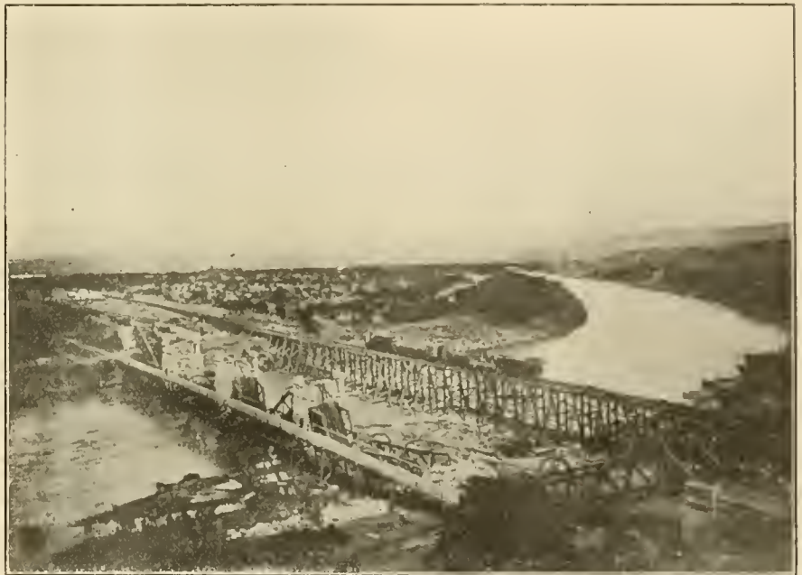
DESTROYED BRIDGE OVER THE COLENZO RIVER, AND TEMPORARY RAILWAY TRESTLE AND FOOT BRIDGE. SOUTH AFRICA.
